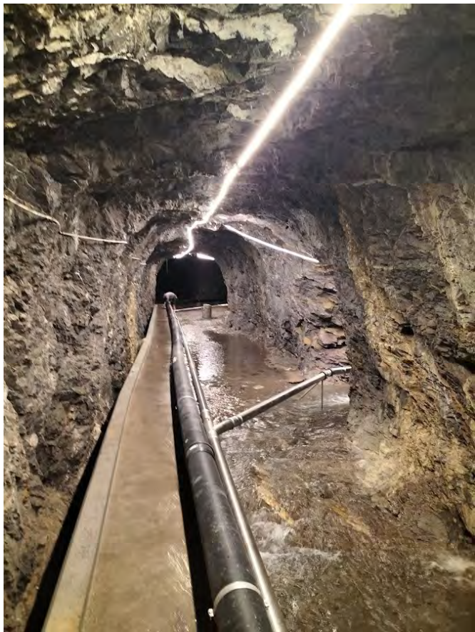
Glarey spring. Collecting tunnel. Supplies drinking water to the municipalities of Conthey. Discharge ranges from 30 to 200 L/s.
