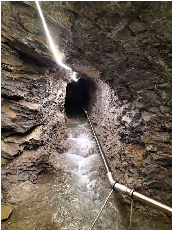
Glarey spring. Collecting tunnel. Supplies drinking water to the municipalities of Conthey. Discharge ranges from 30 to 200 L/s.
